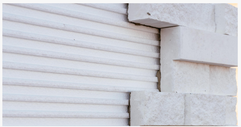
White stone veneer installed on the Stone Panel+ EPS foam panel, showing how the alignment channels support consistent placement and a clean exterior finish.
