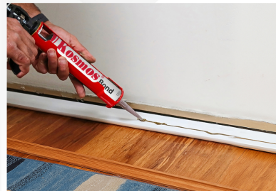
Construction Adhesives Used to create durable bonds that hold heavy loads, replacing mechanical fasteners like nails or screws.
