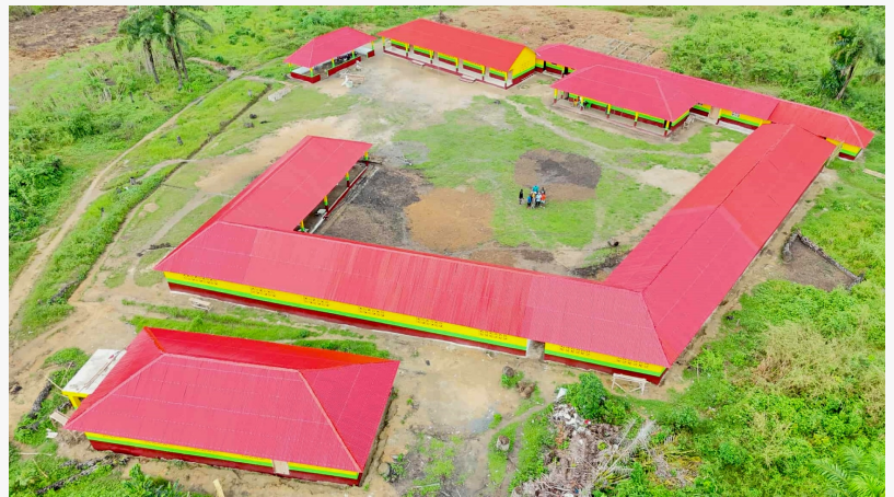
Palm Farm Community School, constructed in under a year through community-driven labor and direct funding
