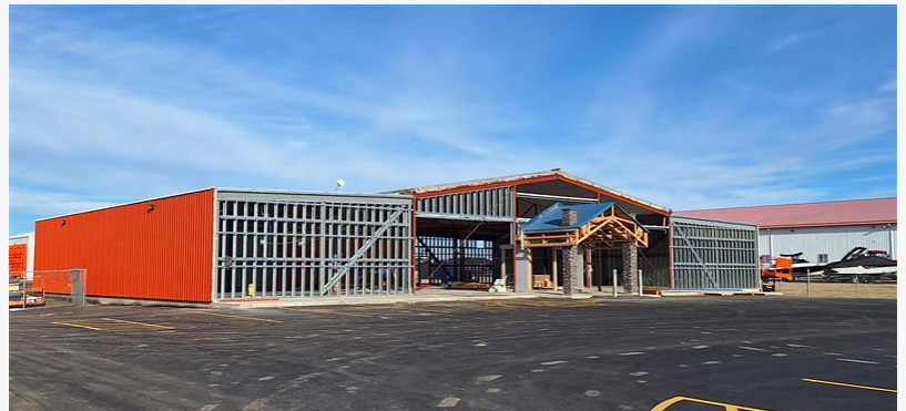
Emerald Park UFA Farm and Ranch Supply Store under construction
