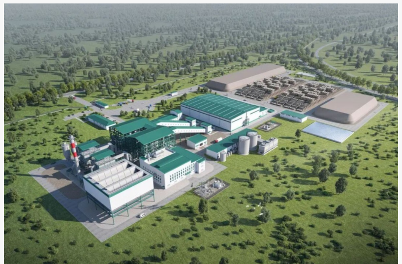
Namibia Biomass Power Plant (Under Construction)
