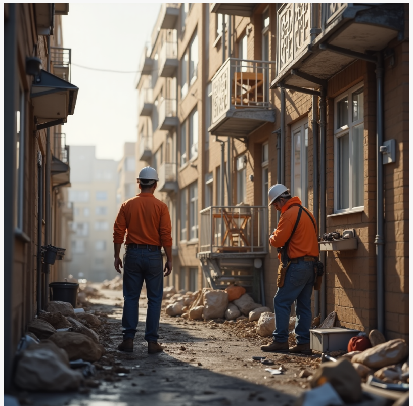
Workers in protective gear carrying out site audits and safety checks on a construction project.
