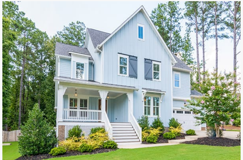
House Painters Prospect
