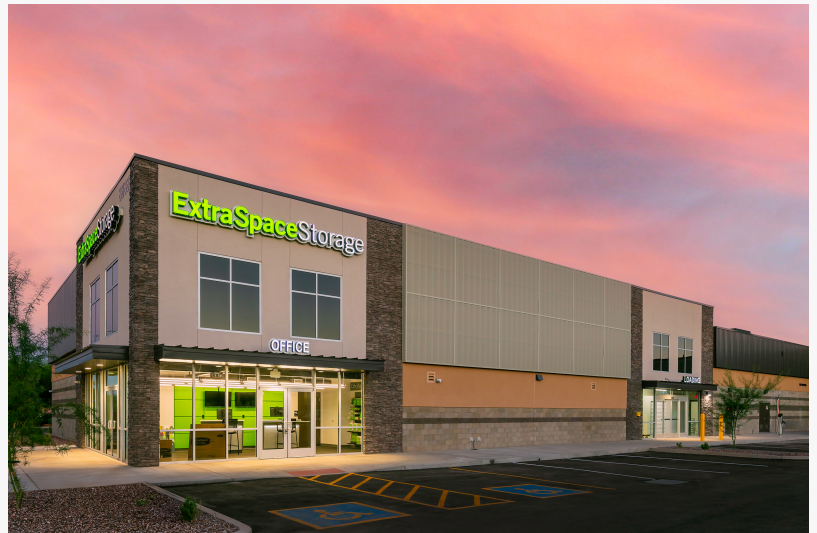
DXD - Scottsdale, just north of the Shea Boulevard and 101 Freeway interchange, this new facility sits in one of Scottsdale's busiest and most convenient corridors.
