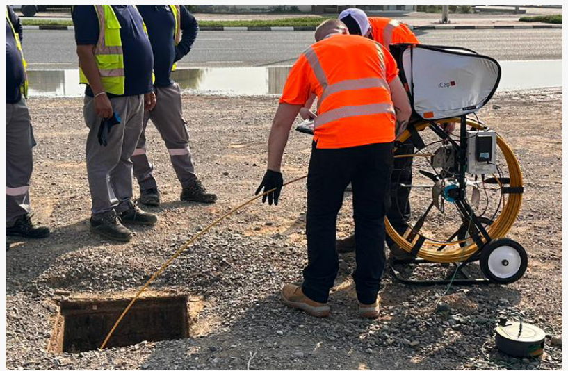
Electro Scan's ES-400 at work for a Middle East client that no longer uses CCTV images to prioritize repairs and rehabilitation decisions.
