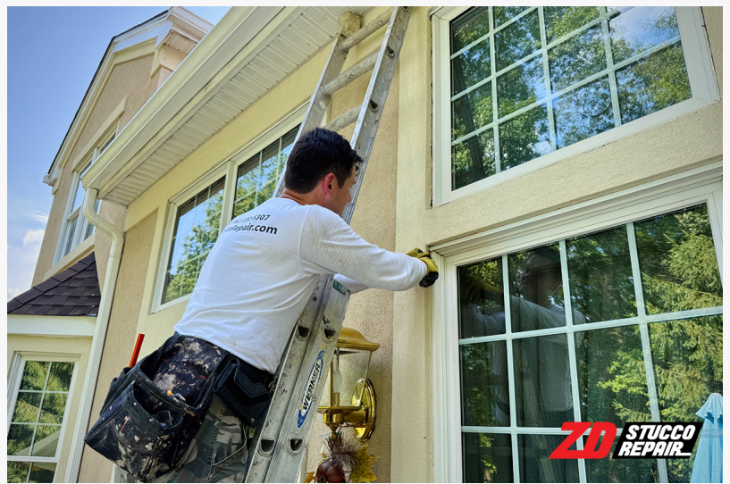
ZD Stucco Repair team member removes old caulking
