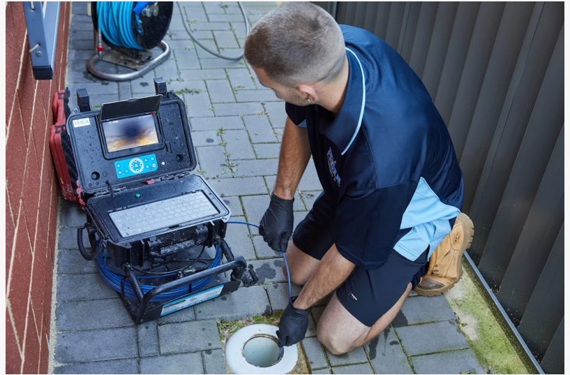
Drain Inspection Proud
