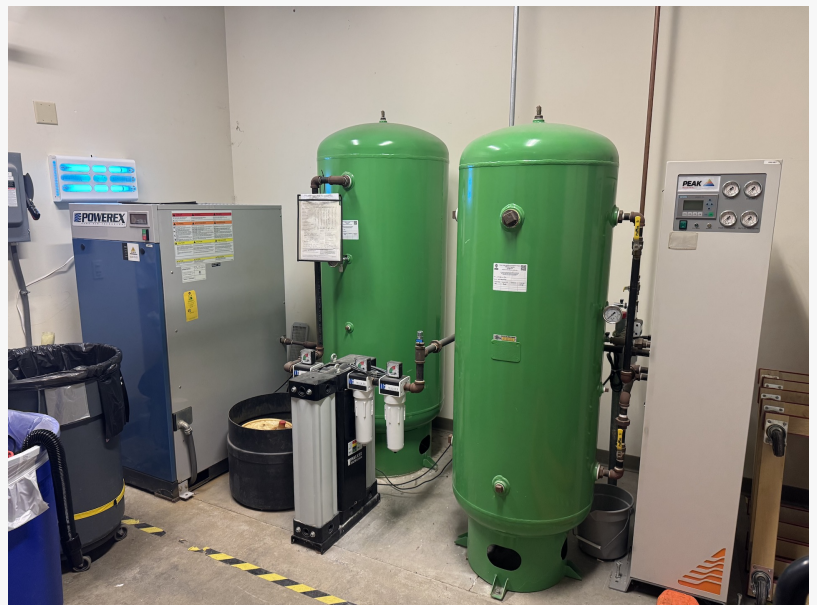
(Lot 93) Powerex SEQ 20-HP Tankless Quadplex Oil-Less Enclosed Scroll Air Compressor and Peak Industrial Nitrogen Generator
