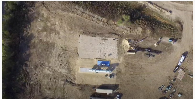
Aerial view of the project
