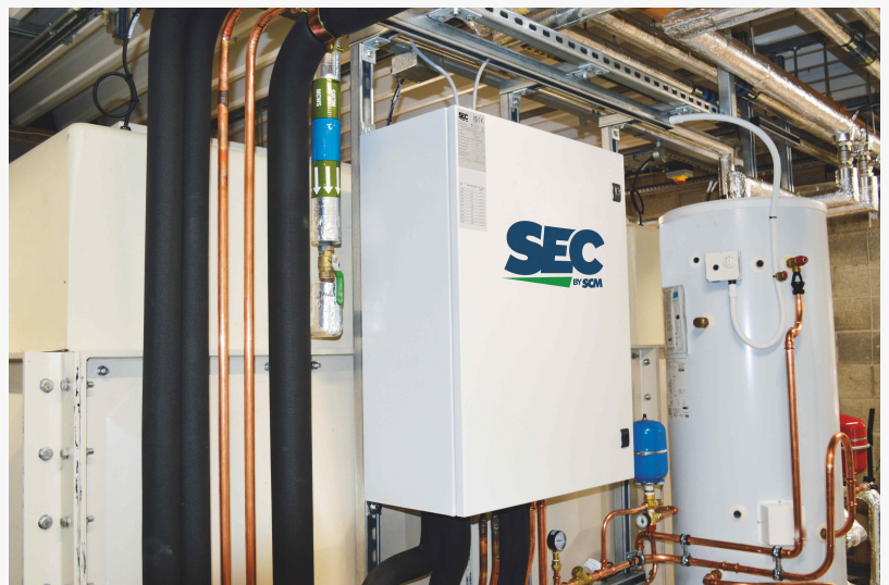
An on-site installation of SEC, providing continuous hot water as a standalone system or from recovered energy from refrigeration systems.
