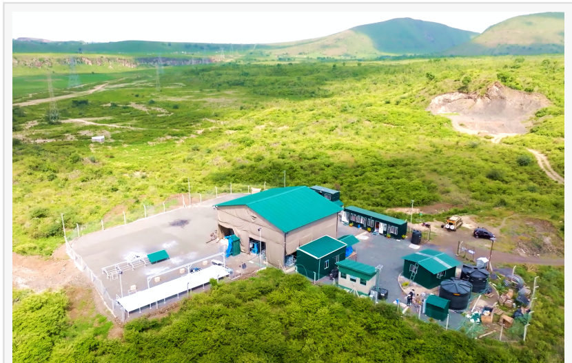
Octavia Carbon's direct air capture (DAC) facility in Kenya
