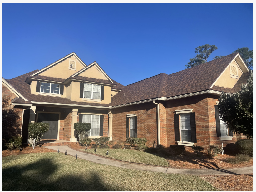
Exterior Painting in Clay County
