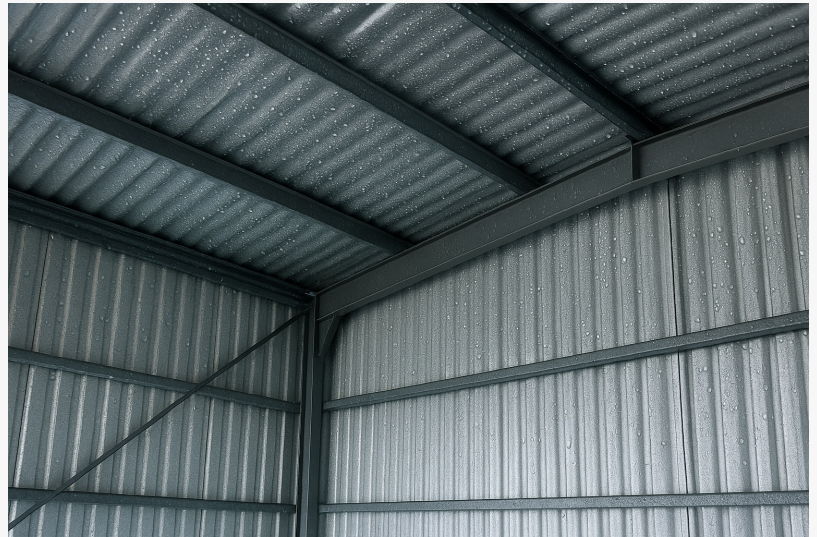
condensation in a metal building
