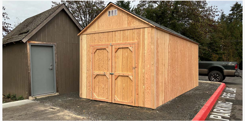
wooden storage sheds
