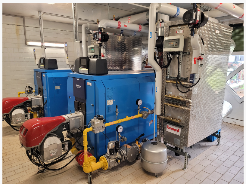
Wastewater facility can take advantage of heat recovery using the BOMAT heat exchange system
