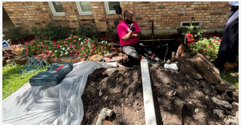
Schedule 40 PVC is the sewer pipe replacement material of choice in DFW.
