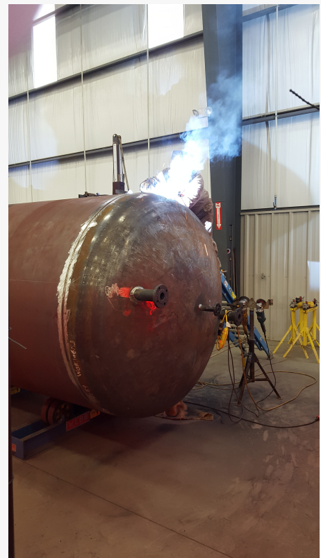
Raw Welding Inc. providing expert welding and fabrication services with precision and care.
