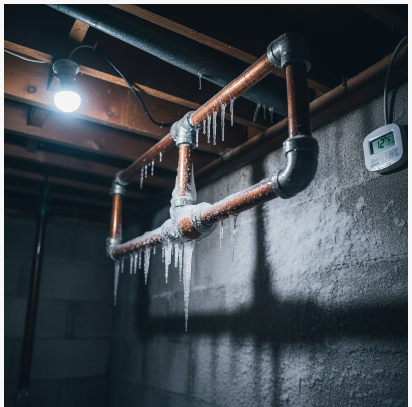
Frozen basement pipes covered in ice and icicles during cold weather.
