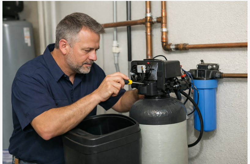
A technician repairing a water softener.
