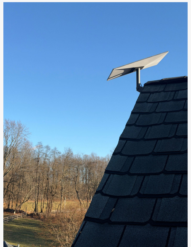
Professional Starlink installation by DishNinjas for residential and commercial customers across the United States.
