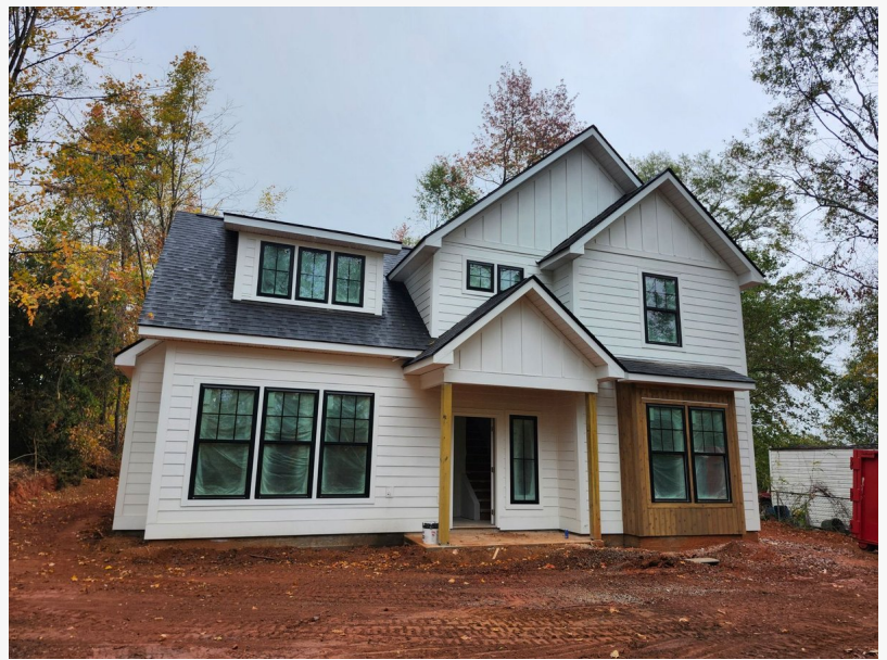
AG Construction Earns Perfect Five-Star Rating in Greenville
