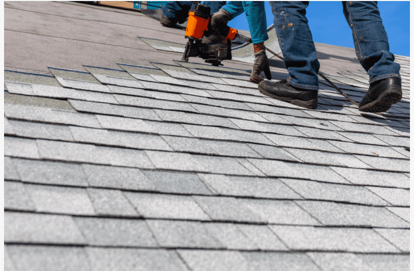
Shingle roof installation underway as part of a residential roofing replacement project.
