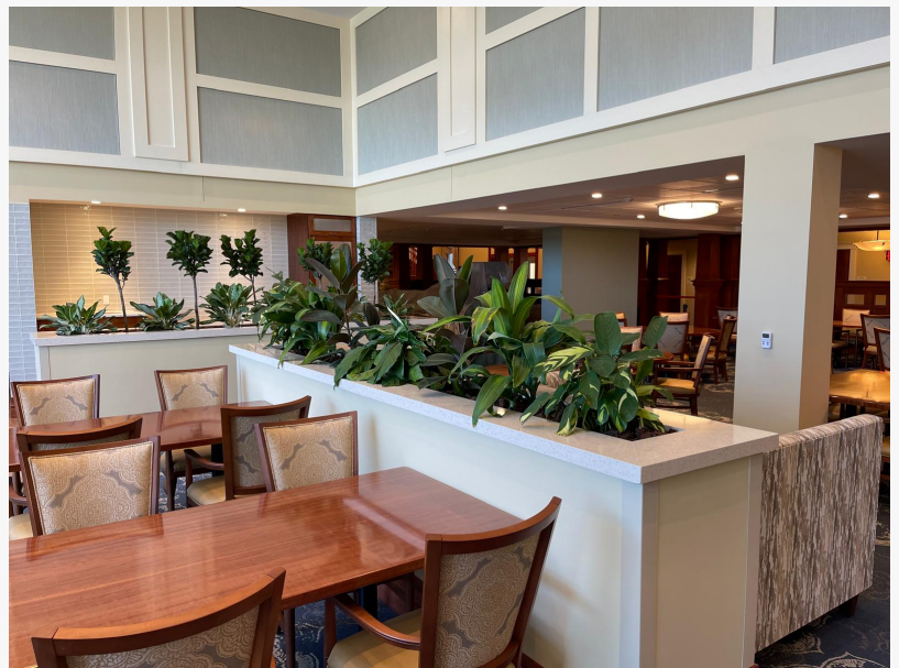
stone countertop fabrication and installation
