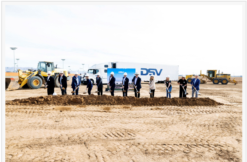
DSV Mesa Groundbreaking
