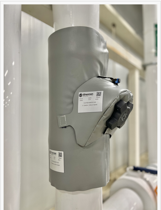
Innovative Shannon Hydronic Insulation Shield on Hot Water Valve helps prevent Heat Loss for energy efficiency in Hydronics Systems
