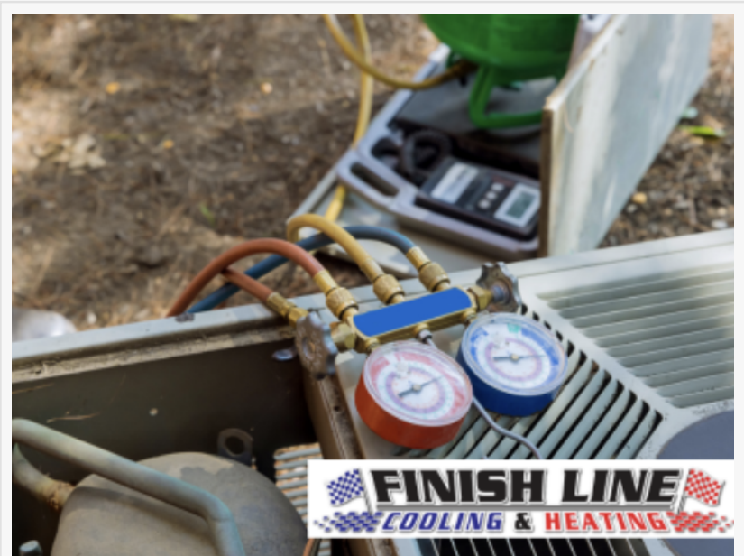
AC Installation And Repair In Venice, FL - Finish Line Cooling & Heating
