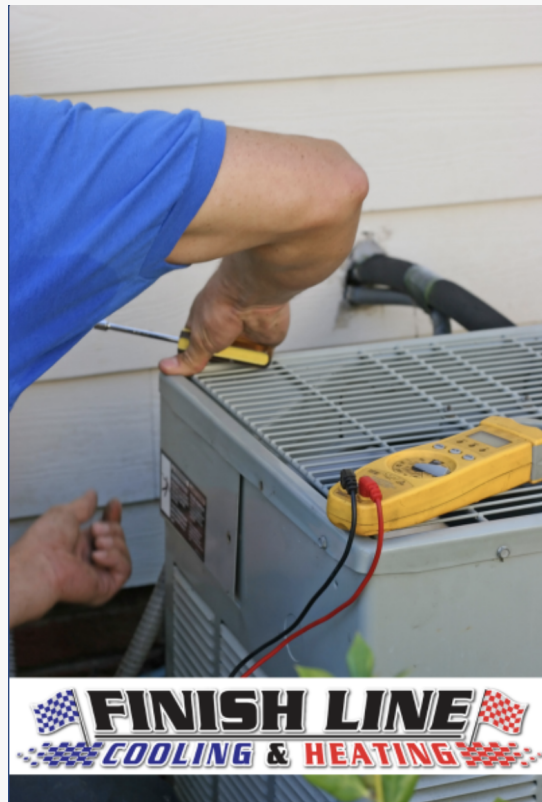
AC Installation And Repair In Venice, FL - Finish Line Cooling & Heating
