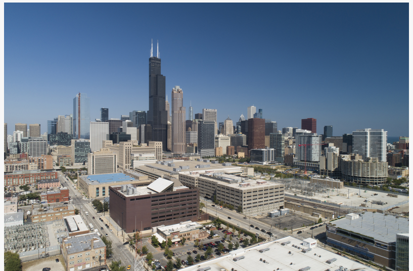
Serverfarm CH1 Chicago Data Center
