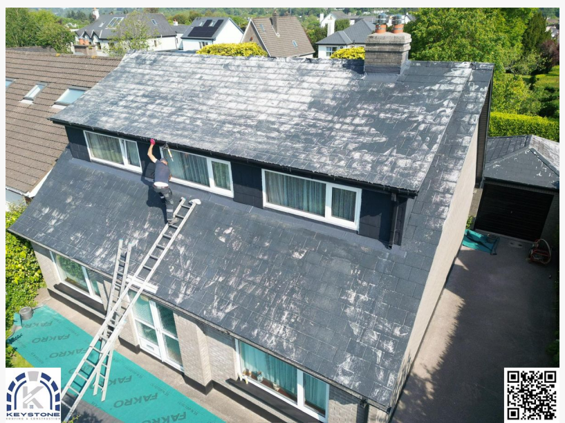
storm emergency roofing service in cork
