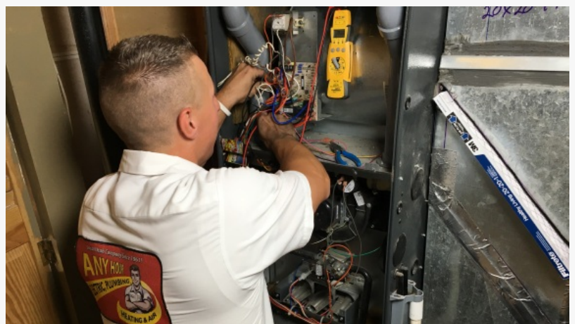
An Any Hour technician repairing a furnace.
