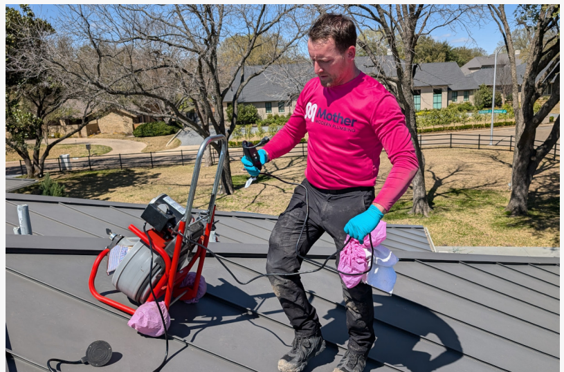
Hydro jetting is the most effective way to remove tree roots from Dallas pipes.
