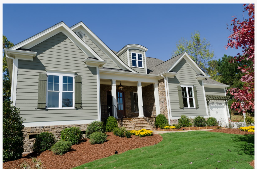
Shingle installation performed during proactive roof replacement planning.
