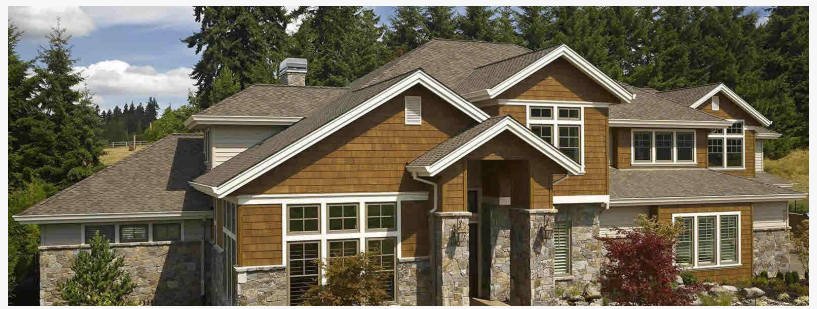
Exterior renovation completed alongside roofing system maintenance.
