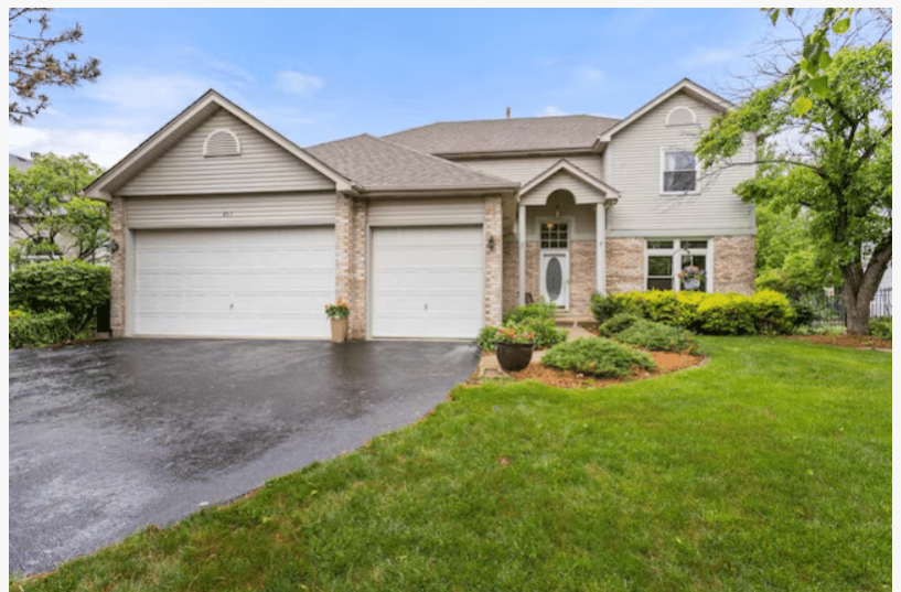
Completed roofing project following preventative restoration work.
