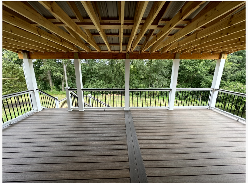
Deck Installer in Beaver
