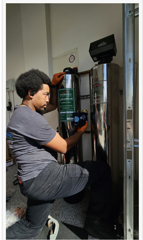
SJ Plumbing Installing Moen Flo Device in Los Alamitos, CA
