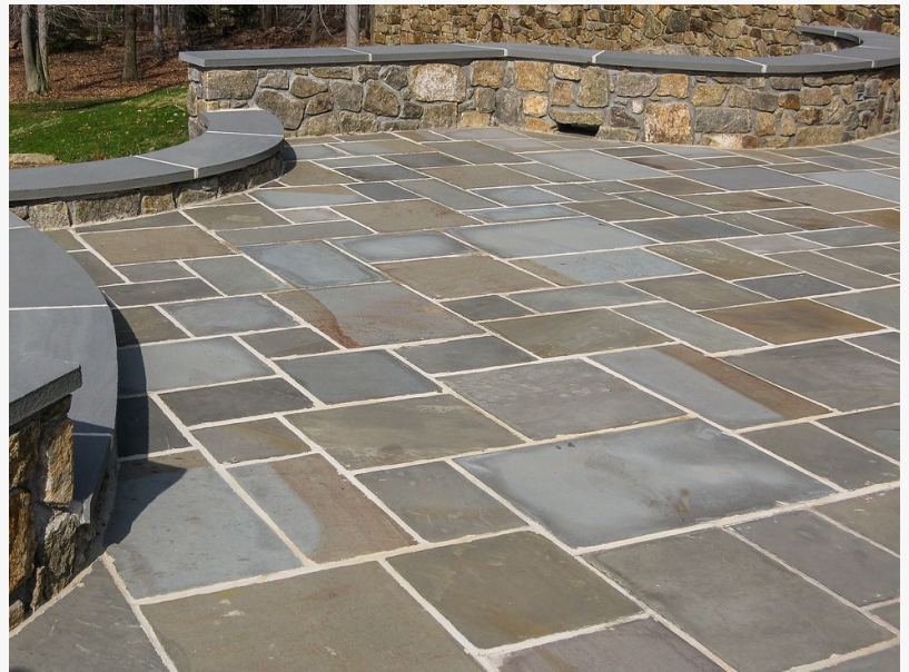
Masonry and Hardscape Construction
