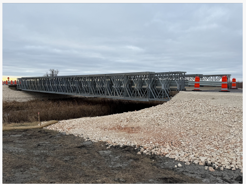
Acrow Bridge in service in Manitoba
