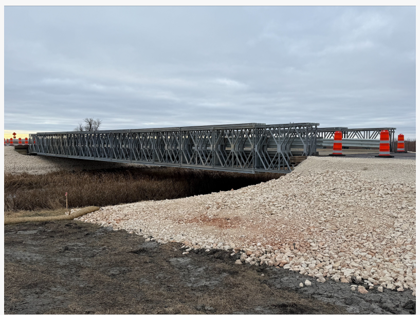
Acrow Bridge in service in Manitoba
