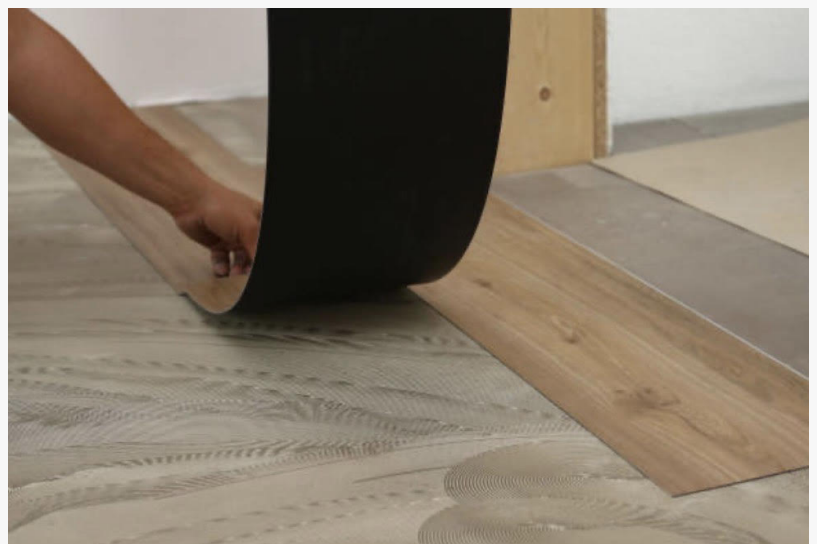
LVT Being Laid
