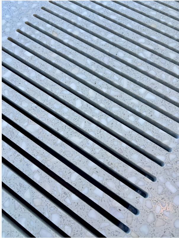
Tiede-Zoeller engineered custom terrazzo air vents to bear foot-traffic.
