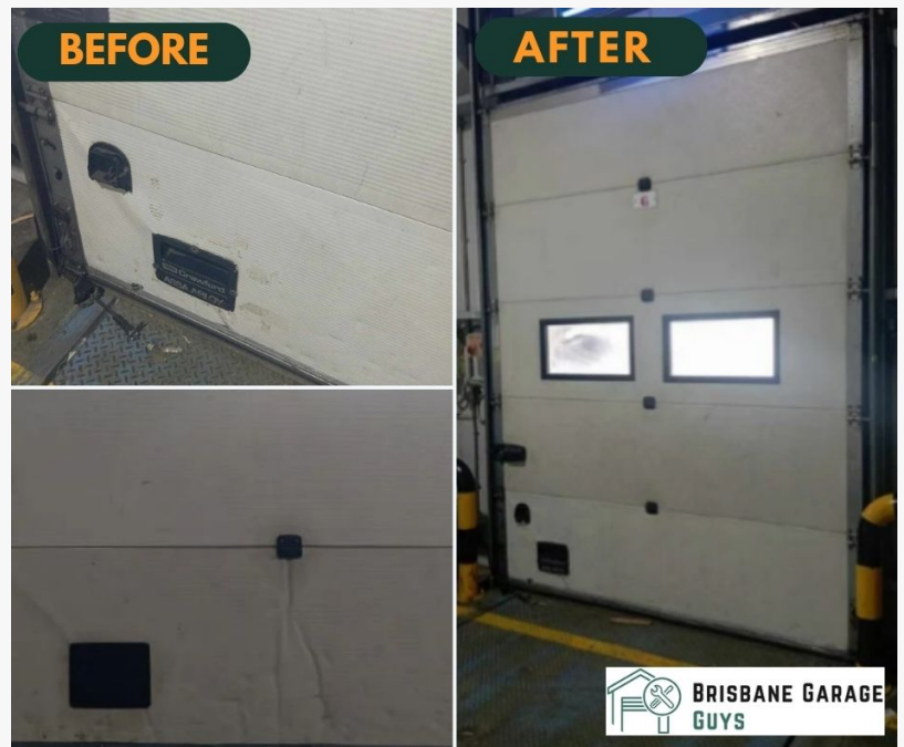
before-and-after-job - Brisbane garage door
