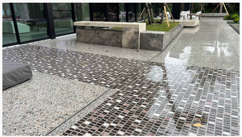
Scarpa Palladiana terrazzo is a focal point of the monochromatic terrazzo installation, bridging epoxy terrazzo interior finishes with a cement-based exterior installation.
