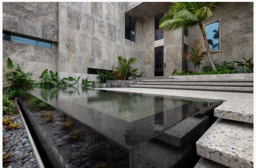
Floating steps leading into the private home in Miami Beach were handcrafted in cementitious terrazzo.
