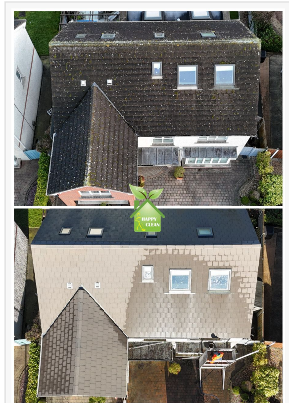
[Before and After] Roof Cleaning Service in Dublin - Happy Clean
