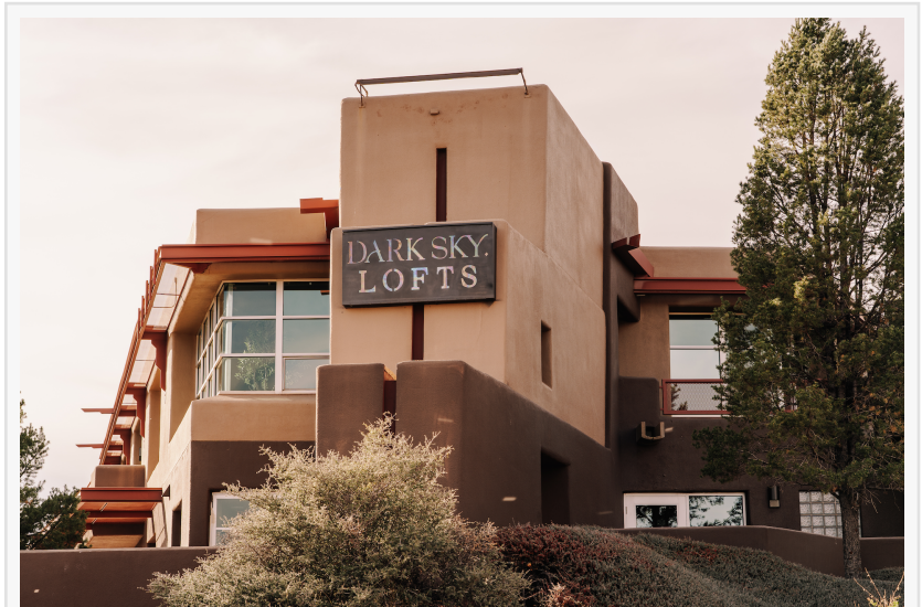
Exterior view of Dark Sky Lofts adults-only retreat in West Sedona featuring modern adobe architecture and luxury loft accommodations.
