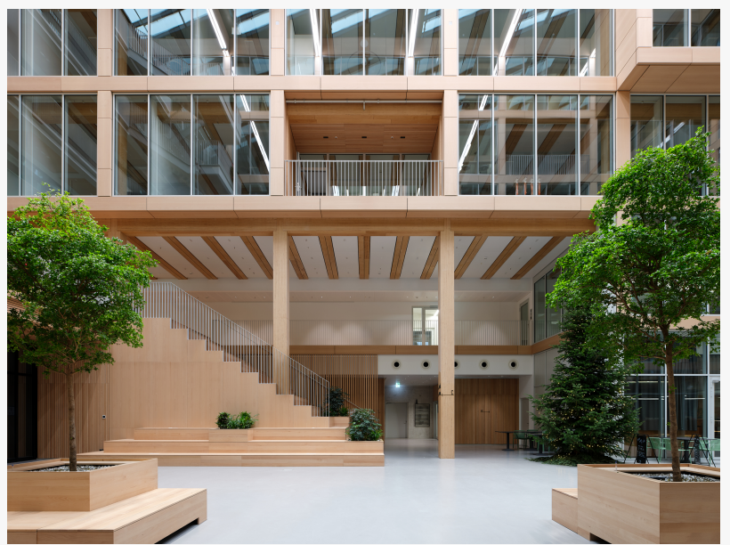
i8 - the green holistic building
