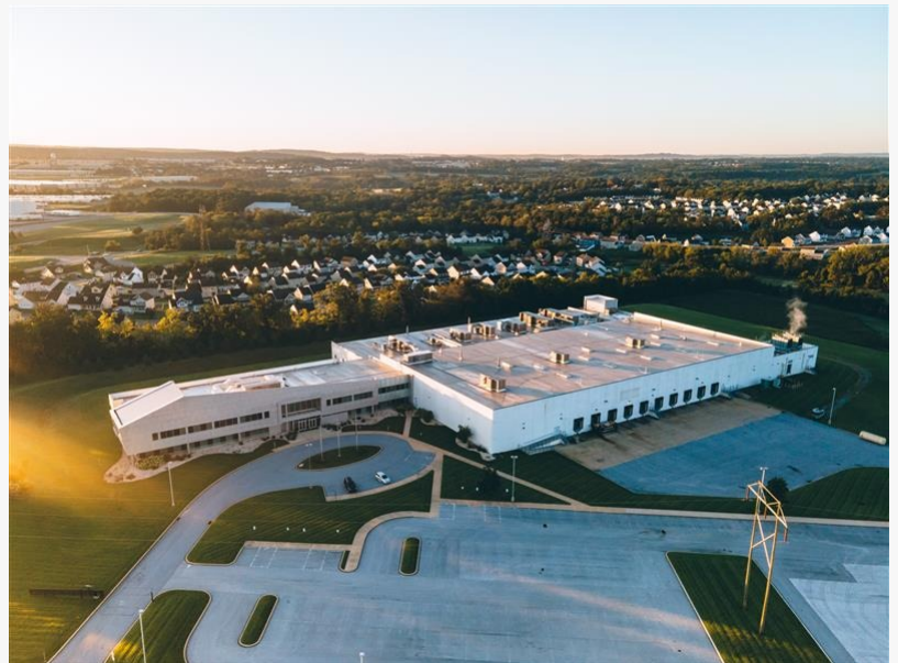
The BioTechnique facility encompasses 268,000 sq ft and sits on 39 acres, with opportunities for future expansion. The facility is equipped with 9 cleanroom suits and advanced manufacturing capabilities.
