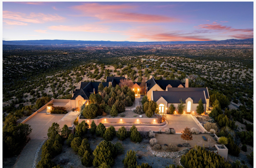
411 Tano Road, Santa Fe, New Mexico
