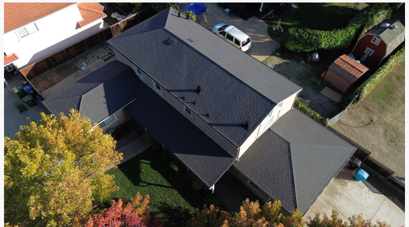
Completed roofing project in san jose ca
