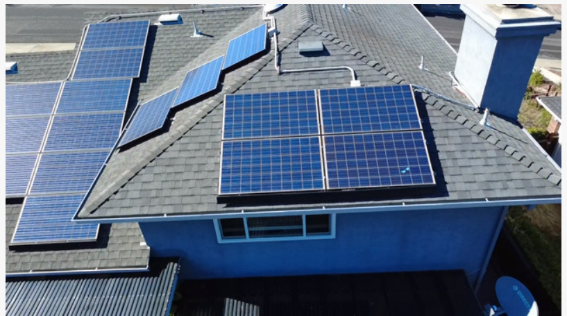
roofing contractors installing solar roof
