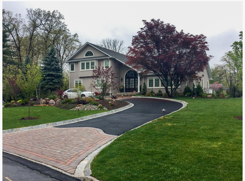
Masonry and hardscape services
